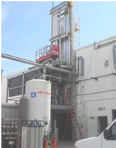
View of 100 mm column installation before weather proofing is added
